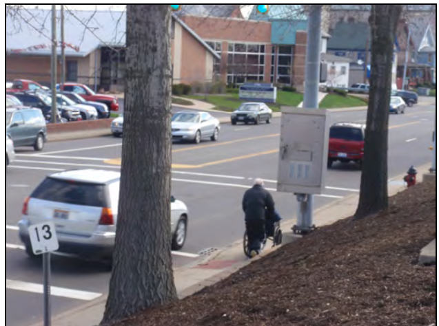
Wheelchair Pedestrian Unable to Reach A Too High Pushbutton
