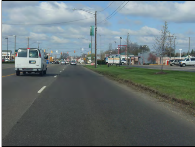
No Curb & Gutter Section East of Whipple
